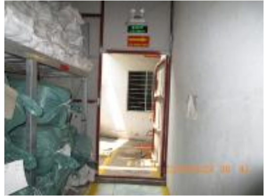
20. Emergency exit is opened outward.JPG
